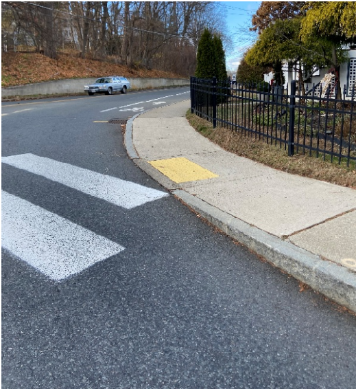
Image 1 - Sight Distance on Finn Street Looking Right
