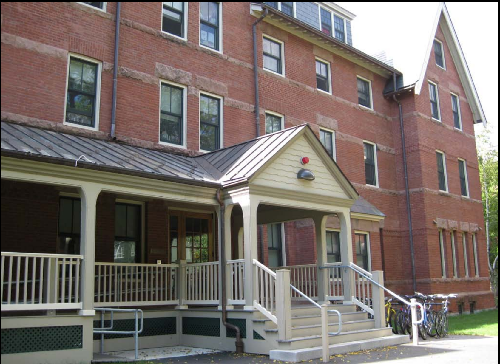
Covered ramp: after
