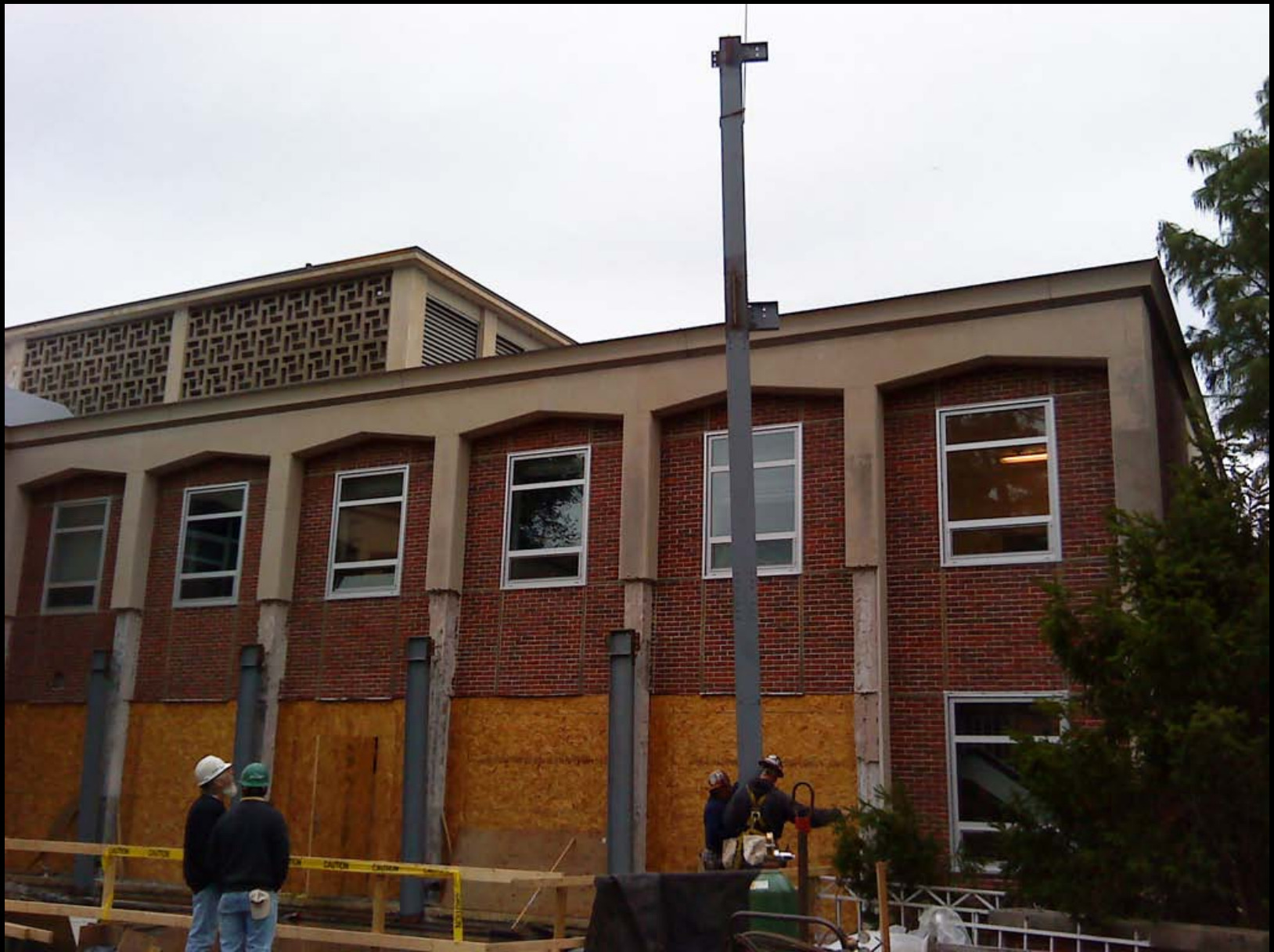
Construction: summer and fall of 2010
