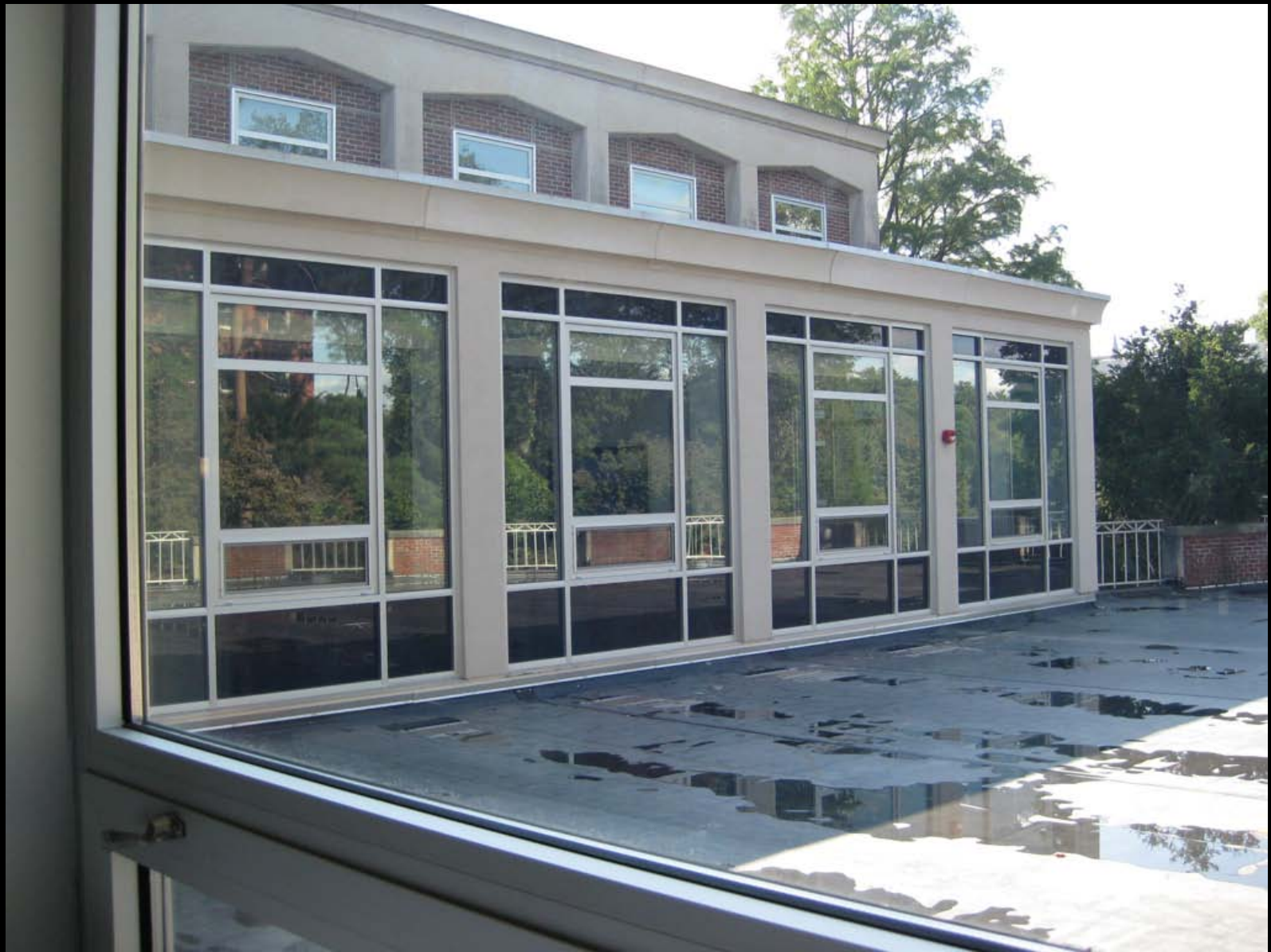
Addition beside terrace for Global Studies Center
