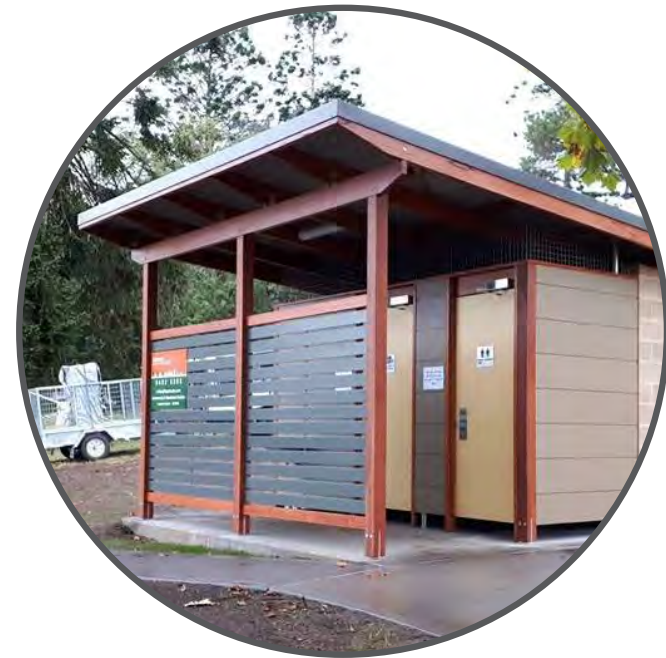
COMPOSTING TOILETS & CHANGING STRUCTURE
