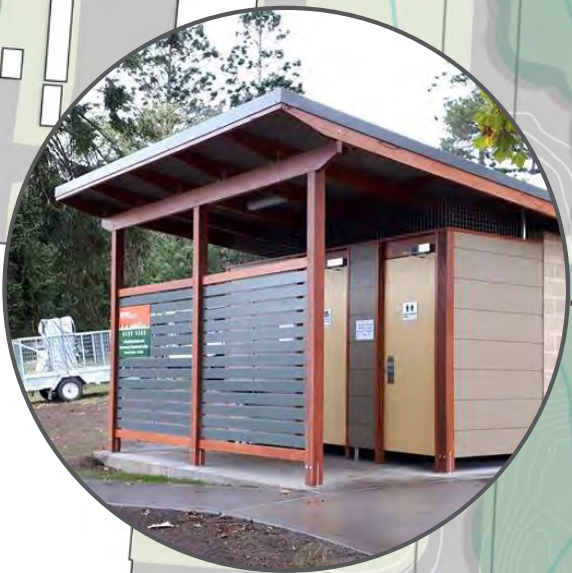
COMPOSTING TOILETS & CHANGING STRUCTURE
