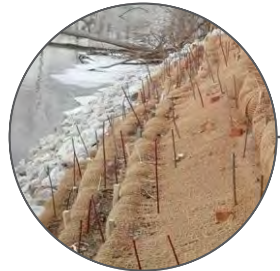
STREAM BANK RESTORATION
