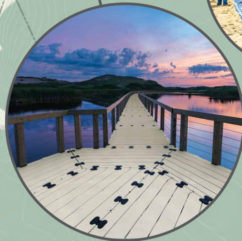
TEMPORARY FLOATING DOCK
