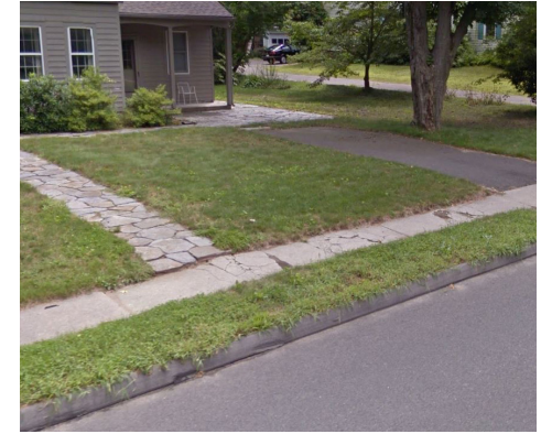
A segment along Prospect Ave that registered the highest pothole count, creating a challenging environment for those with limited mobility. Image: Google.
