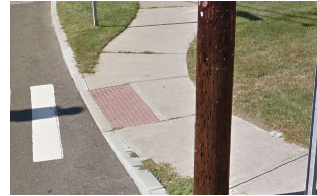
Figure 2.8: A compliant pedestrian curb ramp on Prospect Street at N Elm Street. Image: Google.
