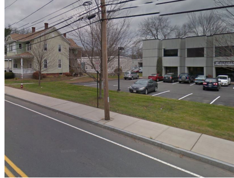
This segment along Conz Street includes utility pole obstructions that narrow the sidewalk width to less than 3' in places. Image: Google.
