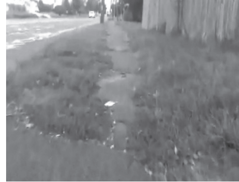
Sidewalk with significant debris in the form of vegetation encroachment, making the sidewalk inaccessible for wheelchairs. Image: screen shot from the rolling wheelchair tablet video.
