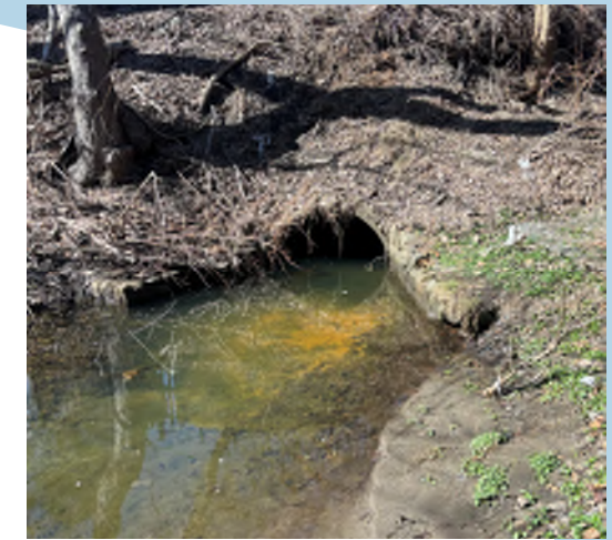
Flooding control area to be dredged
