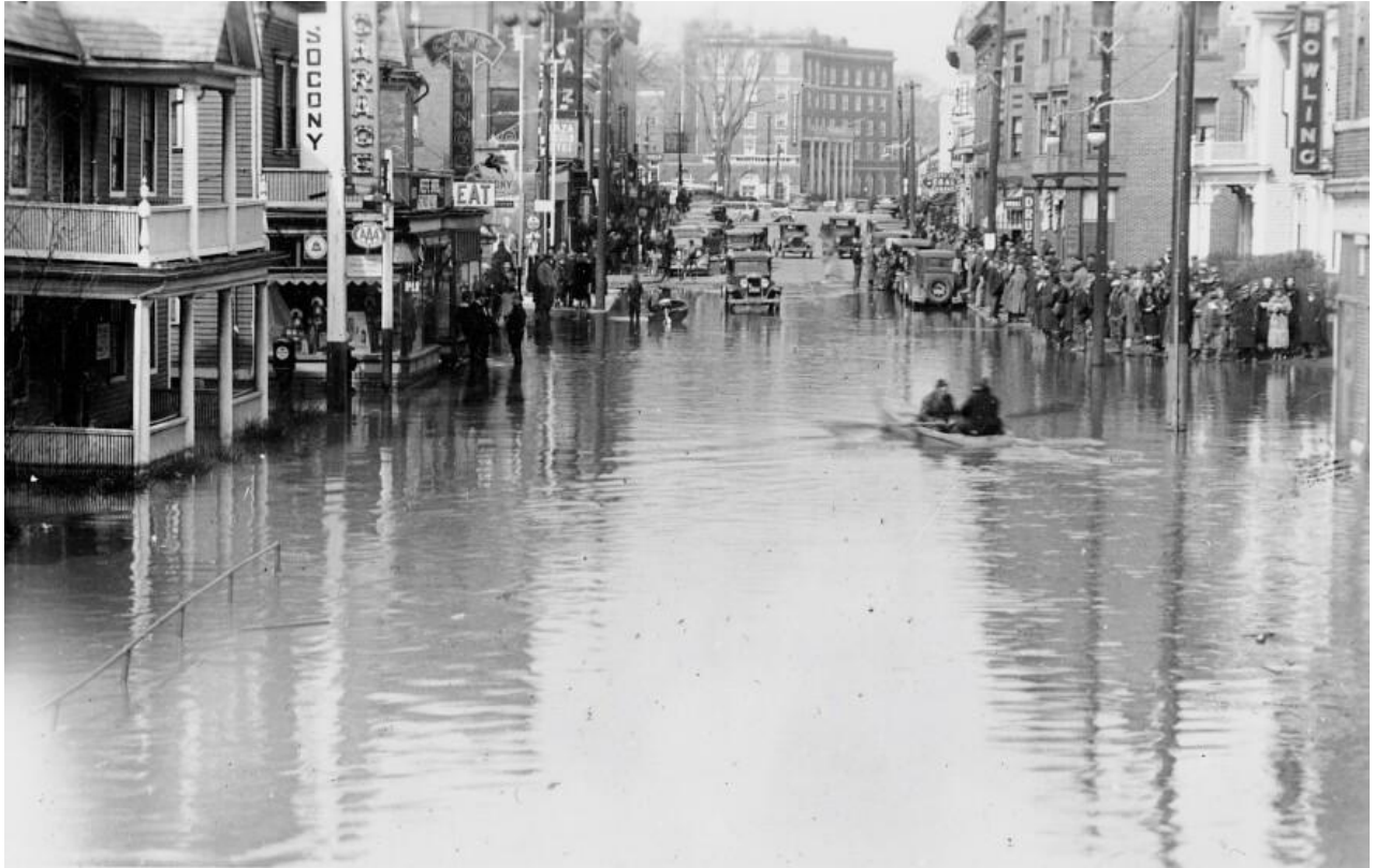
1936 Flood – Pleasant Street
