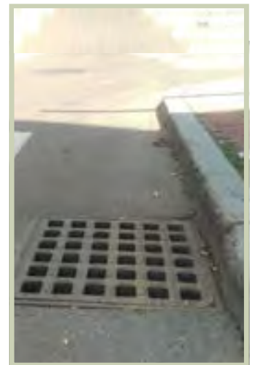
A bicycle-friendly sewer grate in Cambridge, MA. Note the direction of travel and the small opening size.
