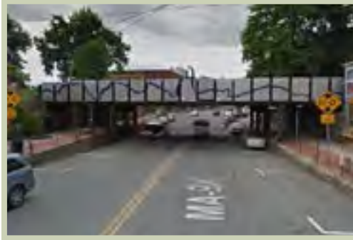
Existing conditions, looking east
