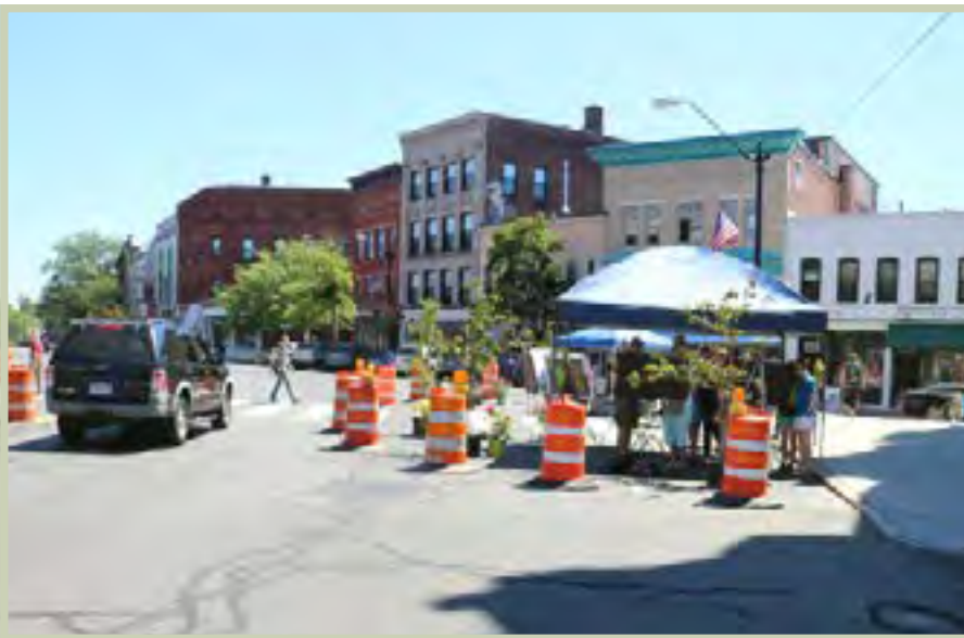
Views of the demonstration project set up that expanded the sidewalk space in front of City Hall and reduced the length of the crosswalk.
