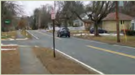
Most sidewalks outside of downtown are five feet wide with grass strips between them and the adjacent roadway
