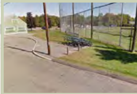
Lack of bicycle facilities & continuous sidewalks along N Maple St. creates a corridor gap between Mass Central Rail Trail, Arcanum Field & Fitzgerald Lake Conservation Area trails
