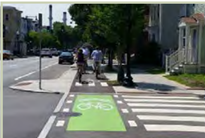
Raised Crossings at Side Streets
